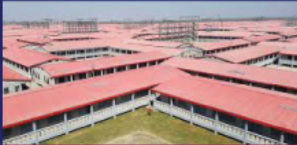
60 x Marineized Shelter Station at Bhasan Char Under Ashrayan Project-3
