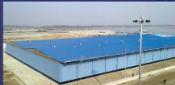
1 x Warehouse for Payra Port Authority (1 Lac. Square Feet)
