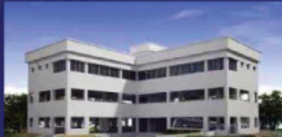
Four Storied High School Building for News Print Mill for MWPGCL at Khalagat, Khulna
