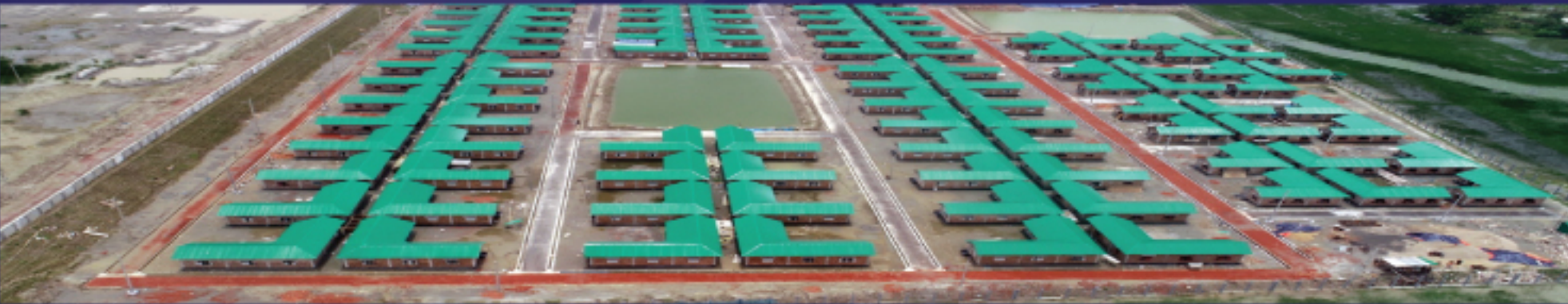
Rehabilitation & Resettlement works under Payra 1320 MW Thermal Power Plant Project
